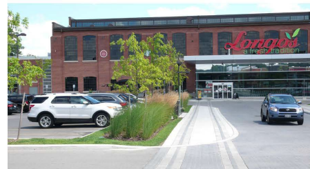
Walkways and landscape divide large parking areas.
