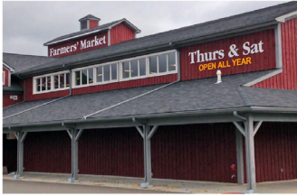
> Clerestory with window band of separate windows.
