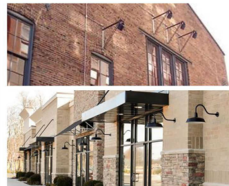
> Decorative exterior building-mounted light fixtures that illuminate signage or pedestrian areas.
