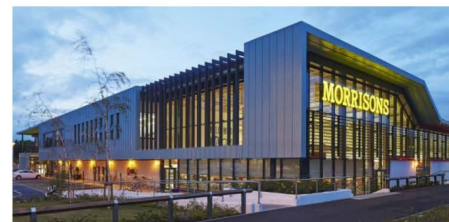
Walkways to building entrances.
