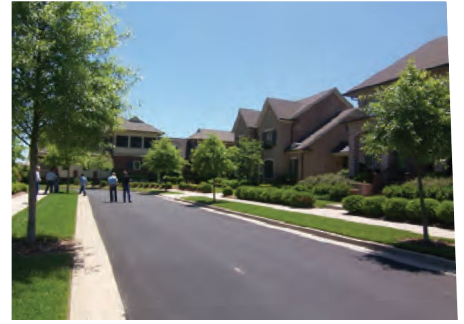
Residential units define the street edge.
