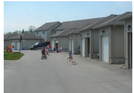
Utilizing lanes for more than garage access.
