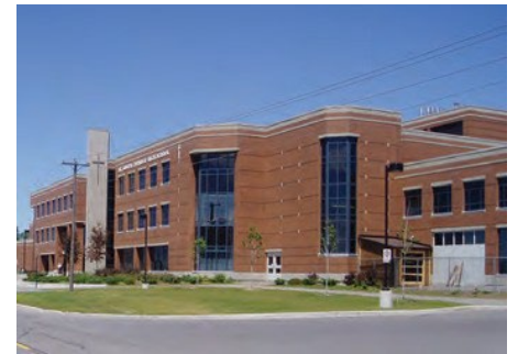
School reinforcing the road edge
