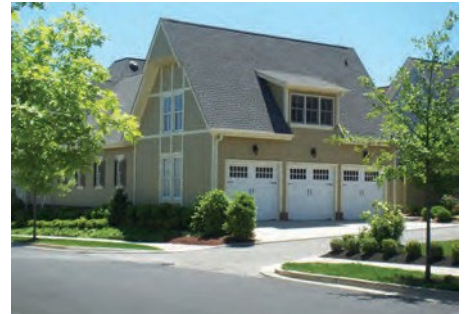
Attached rear yard garage accessed by a laneway
