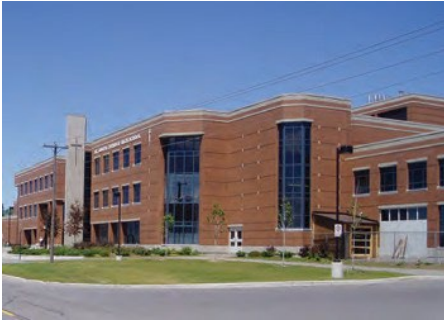
School reinforcing the road edge
