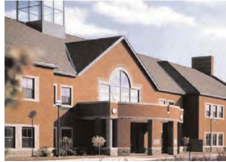
Projecting entry and tower element emphasize the main entrance
